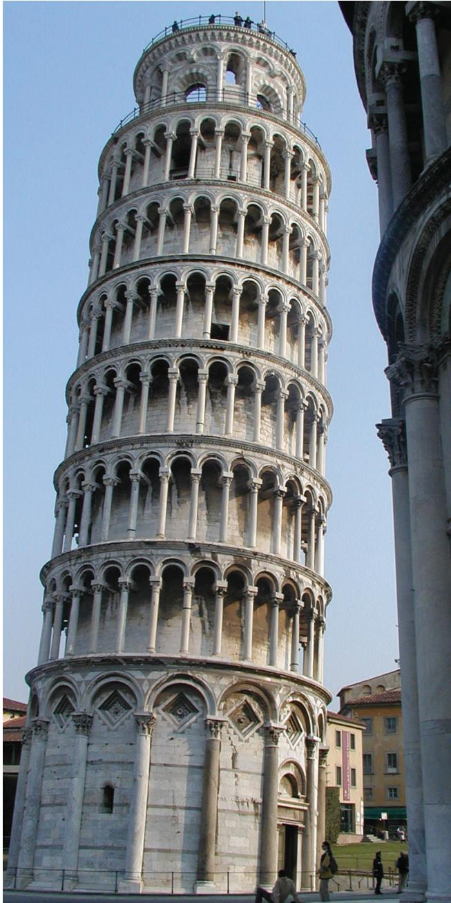
ing, so the tower was closed down and an expert team began carrying out a project aimed to stop the large increase in inclination and try to slightly correct it. The project lasted for about ten years and ended in success. The tower was moved back by half a degree and its inclination rate was considerably reduced.
